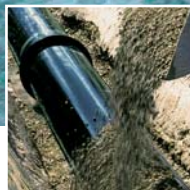
Fast and economic pipe-laying
