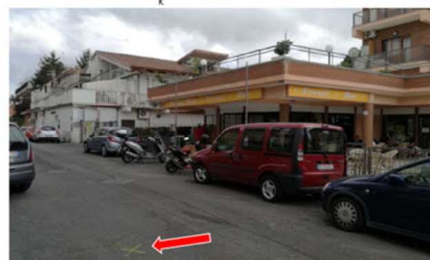
Leak in main line on Via dei Bentivoglio near no. 30
